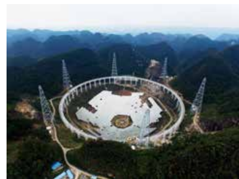
索网结构及反射面单元安装 Cable-net structure and installation of reflector units
